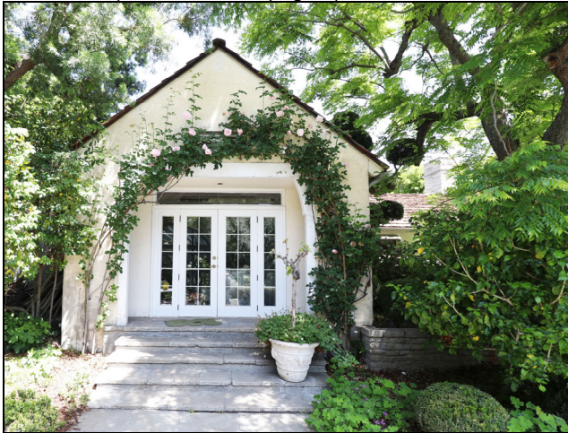
South elevation of enclosed patio on the southwest end of the rear elevation. View north (5/6/22).
