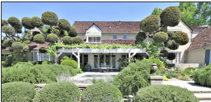
Partial view of the south (rear) elevation and non-original trellis in front of the loggia, view north (5/6/22).
